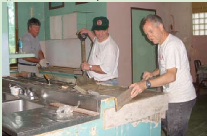
Carl, Marv and Mike pouring concrete countertop to foil the termites
