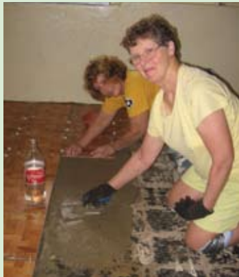
Marlene and Gerry laying tile
